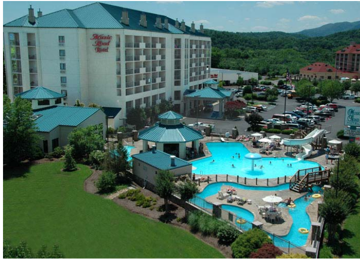
Fig. 4. The 162-room Music Road Hotel in Pigeon Forge, Tennessee, agreed to host test DSI's controllers providing spinning reserve.
